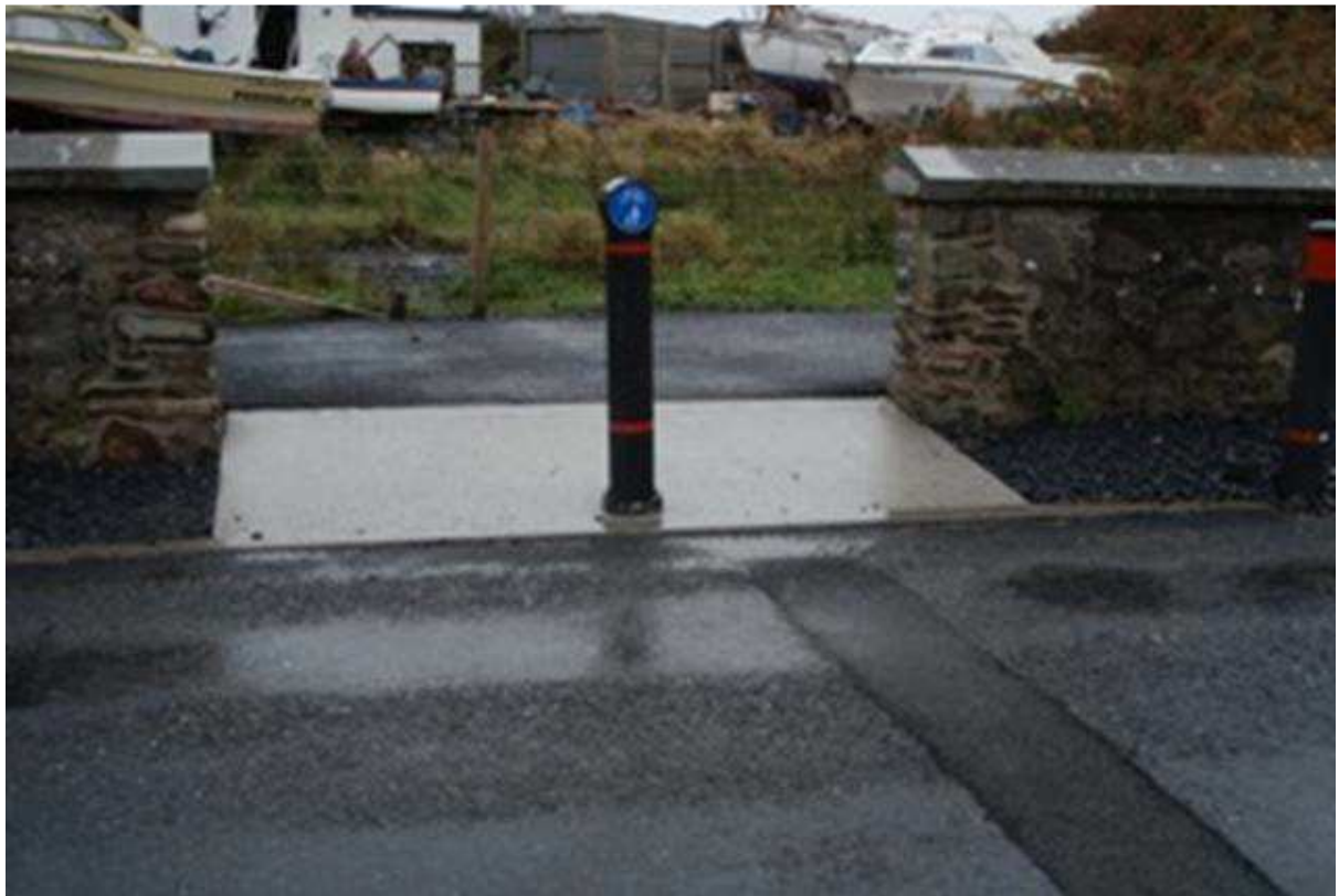
Lagavilin exit on to road
