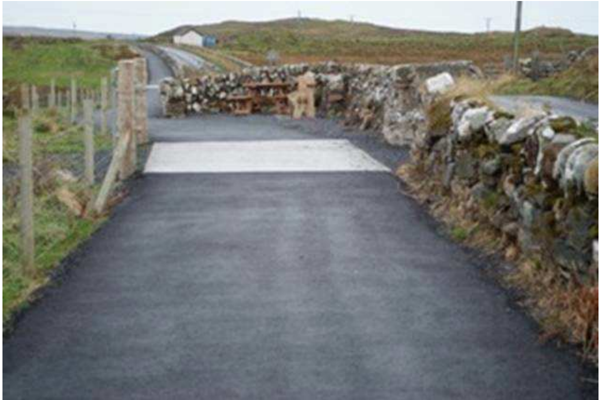
Farkin hill looking towards Port Ellen with Colas surface
