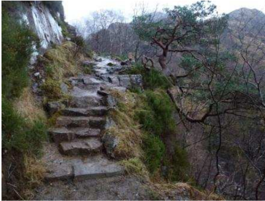
After - stone steps built over tree roots to protect them
