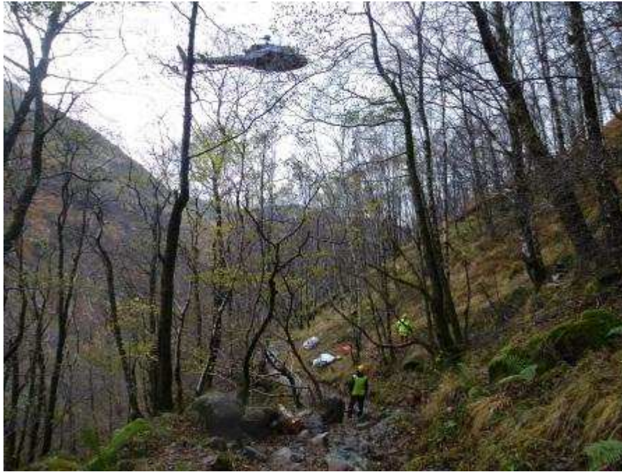
Helicopter landing bags of stone on a long line
