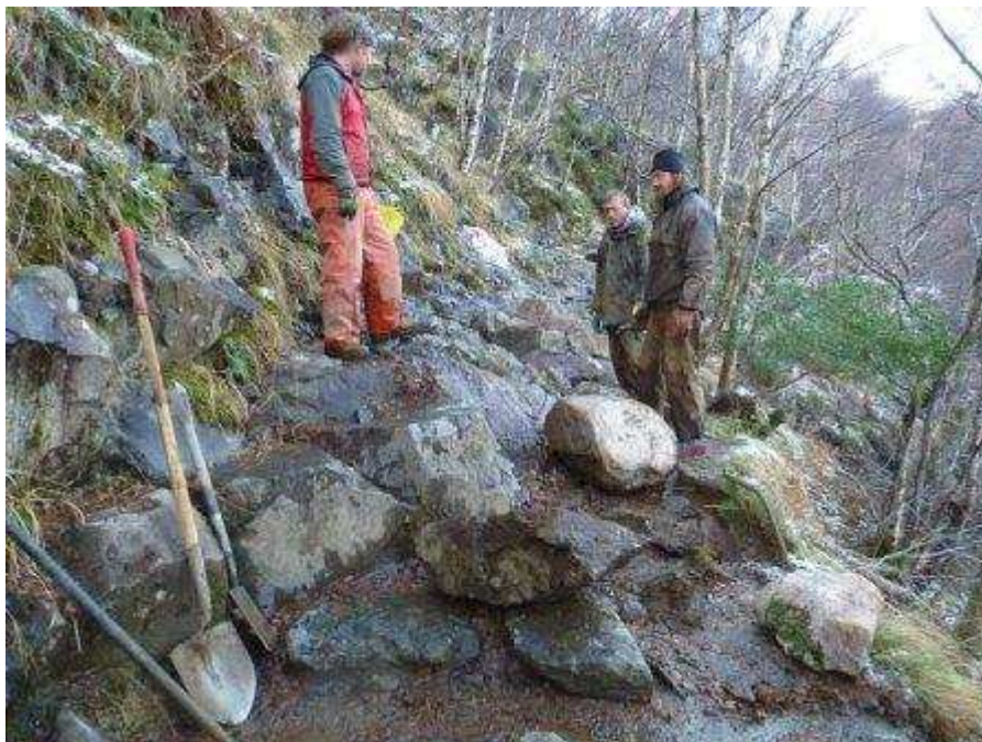
Before - awkward bedrock section with braiding on the right hand side
