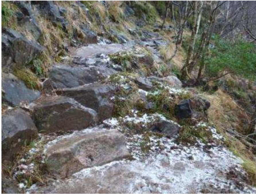
After - revetment veins landscaped
