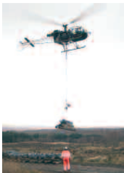
Lifting heavy materials by helicopter allows fencing to take place in otherwise inaccessible locations.
