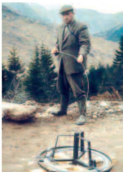
Some aspects of fencing have not changed over the decades; here running out line wire that will support hinge joint netting.
