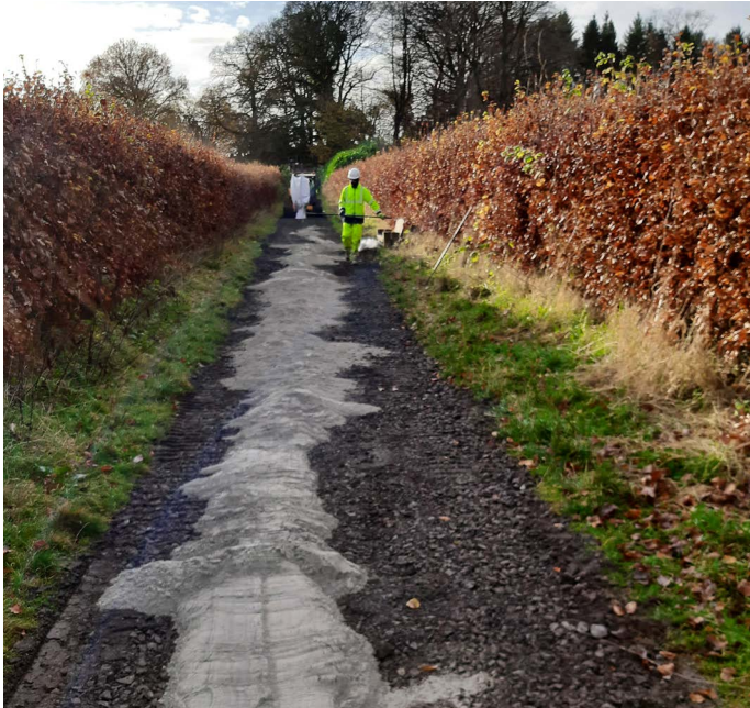
Figure 2 – Smart Surface powder being dispensed over the specified area
