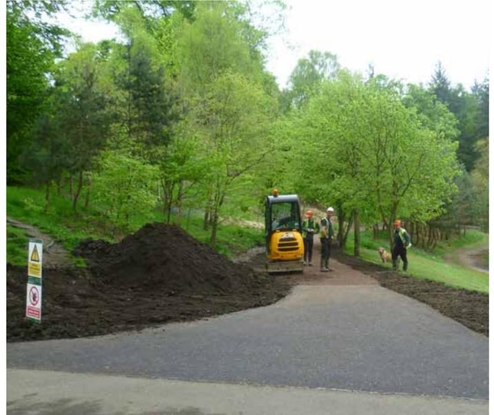
Transition zones between the new path and existing tracks through the wood needed particular attention to maintain the right gradient.
