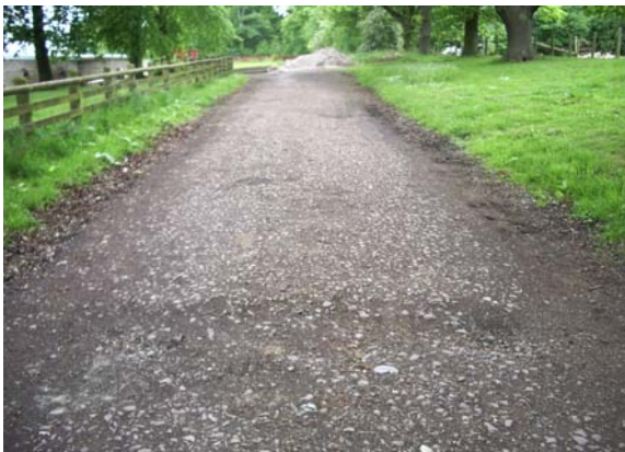
The old path breaking up and the new laid surface.
