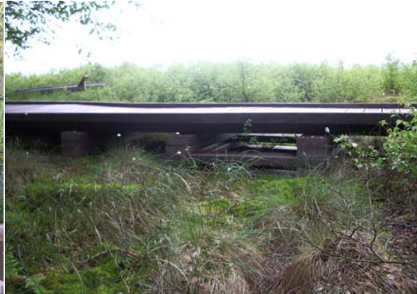
Floating bridge endseats and floating boardwalk.
