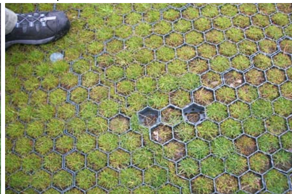
The Gopla grass reinforcement system.
