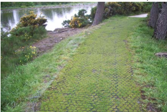
The Gopla grass reinforcement system.
