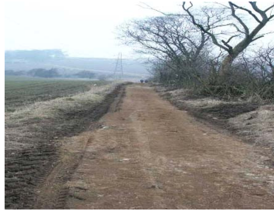
Newly completed path.
