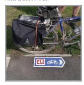
Figure 24: Preformed thermoplastic marking on traffic-free section of National Route 45, manufactured by Preformed Markings SW
