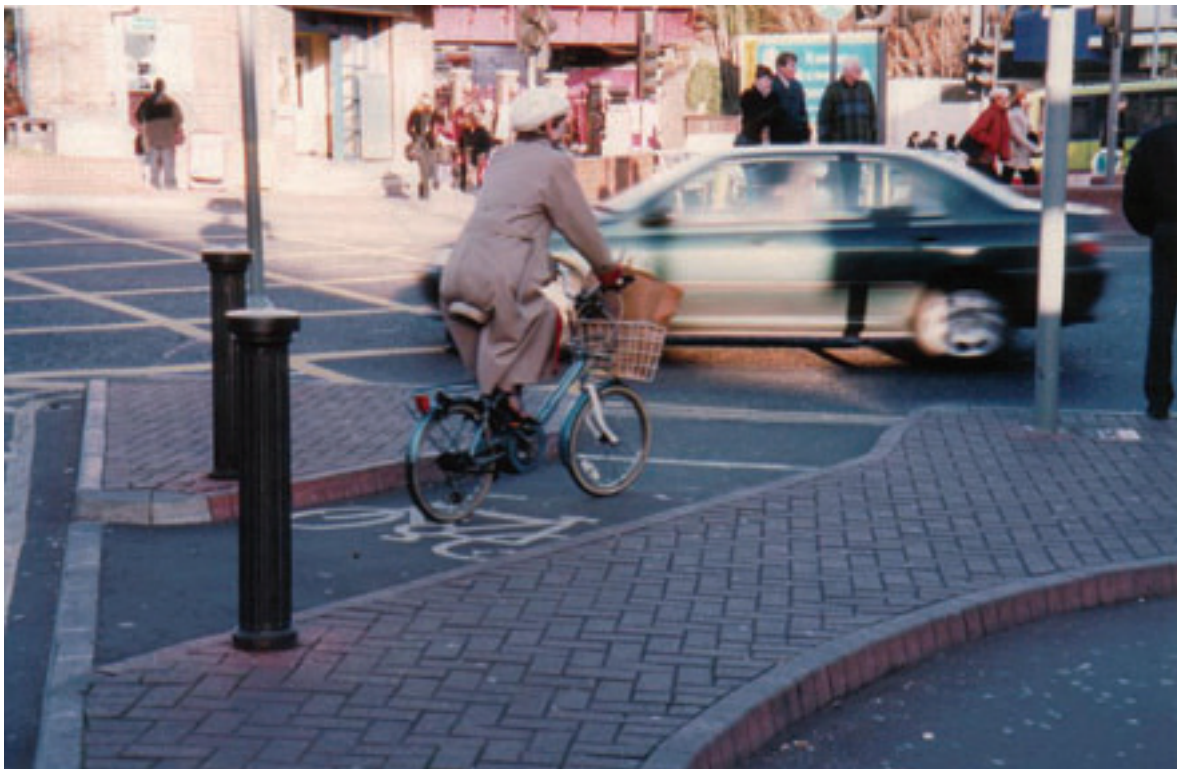
‘Fast’ junctions can be made much safer for cyclists, like this one outside Kingston-upon-Thames railway station
