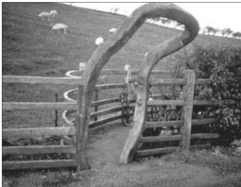
The "wind-blown gate", an access control designed to contain livestock and deter illegal motorcycle use while permitting walkers, cyclists and wheelchairs. Access controls need not be of uniform design and so can be designed to be visually interesting and appropriate to the location.
