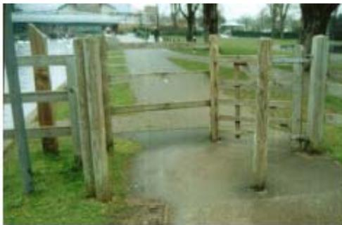
These examples no longer perform the function for which they were originally installed. Gaps within or adjacent to the barriers mean they no longer restrict motorcycle use
