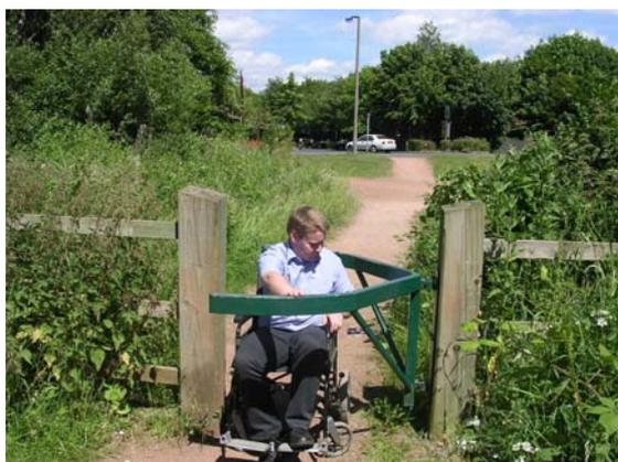
The gate pivots on a central hinge and allows wheelchairs through but motorised buggies will experience difficulty.
