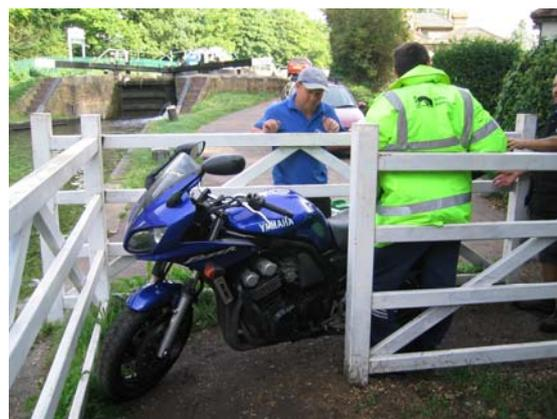
Has the appearance of conventional wooden gates but made of steel. Allows motorised buggies through. A third barrier can be added to further impede trials bikes. The height makes it very difficult to lift bikes over.
