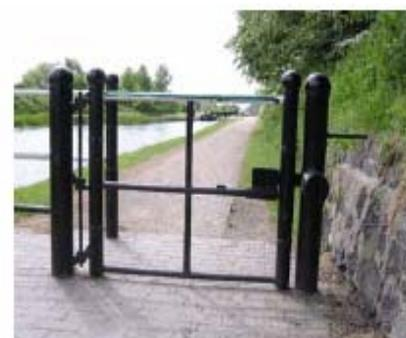
Gates across the canal system also vary enormously. The key factors with respect to their accessibility for disabled people relate to their opening width and direction and whether they have latches or locks. Gates with latches that are easily used from both sides and that open both ways are likely to be less restrictive. The need for a gate rather than a gap should always be questioned.
